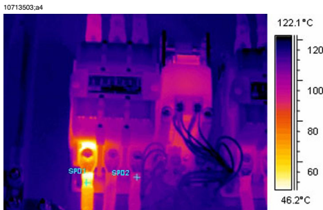
Figure 13.9 An infrared image of indoor electrical equipment (2)
